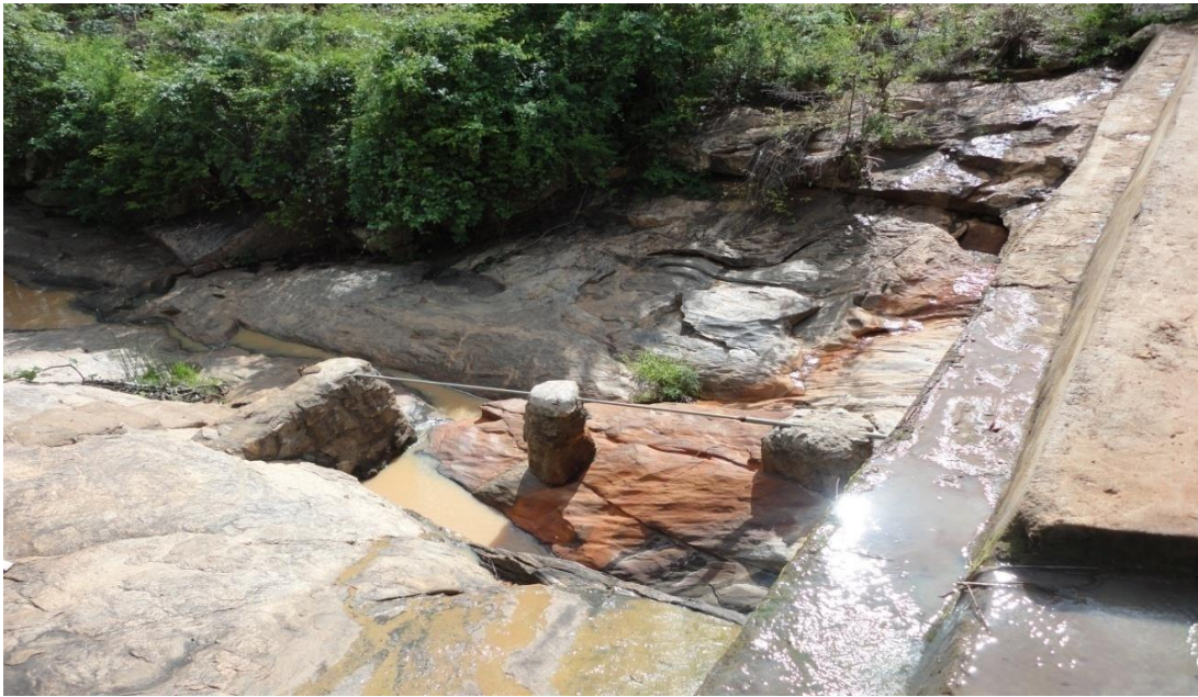
Plate 2: Subsurface Dam with gravity-pipe at Ilalambyu, Kitui County, Kenya
